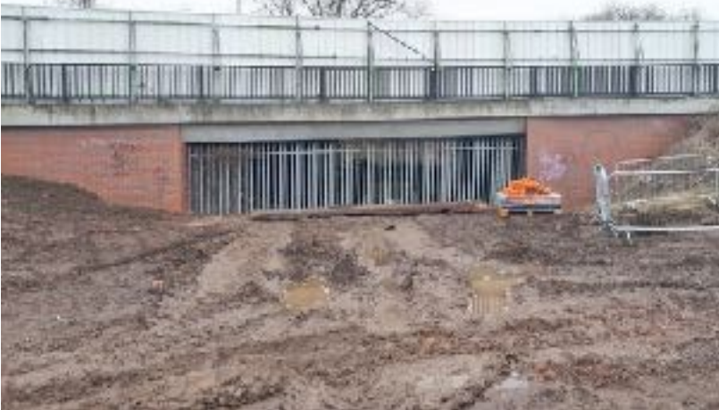
Photo 3 Construction of undercroft under the goods delivey yard
