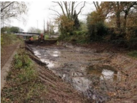
2000 cubic metres of soil removed
