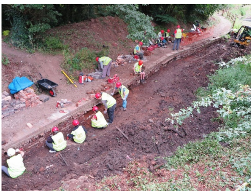
Starting on repairing the wall
