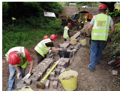
Repairing the top of the wall
