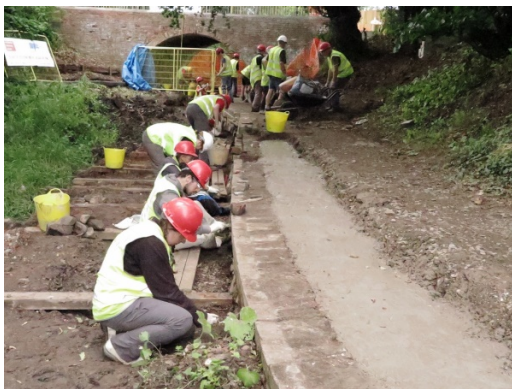
Ongoing wall repair
