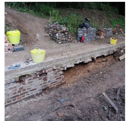
Repair in progress
