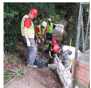
Building a retaining wall for the access path
