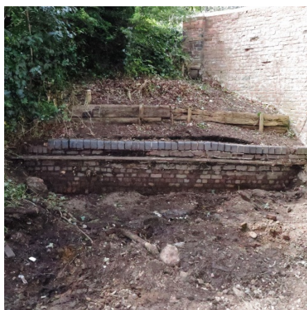
Uncovered offside wall in good condition
