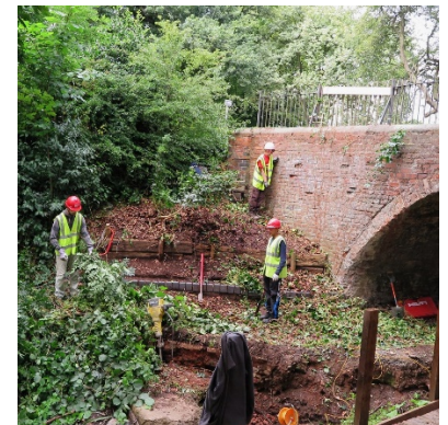
Removing vegetation damaging the bridge
