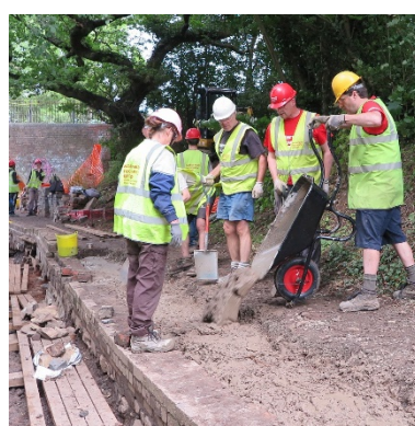
Pouring concrete for wall support
