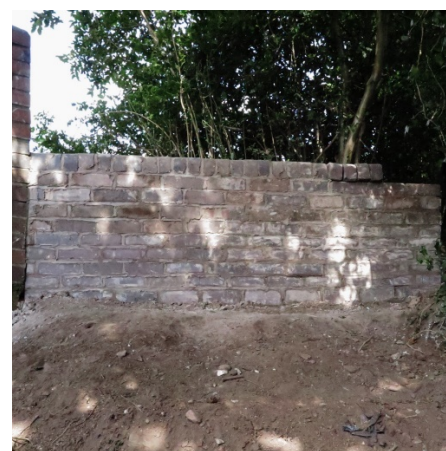
Access path retaining wall using old bricks
