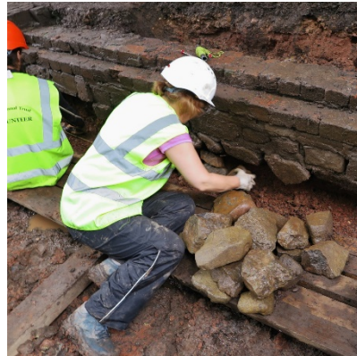
Carefully reassembling the stone foundation
