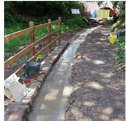
Finished concrete support wall
