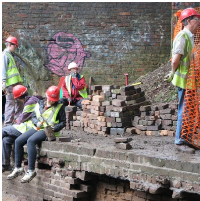
Busy cleaning bricks for reuse
