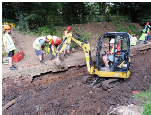
Clearing the wall
