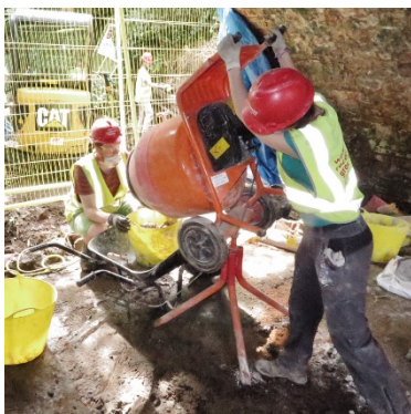
Mixing the large amount of cement used
