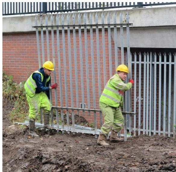
Reinstalling the Tunnel Safety Fence
