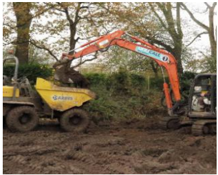
Careys removing the soil from Harborne Wharf Nov 2015
